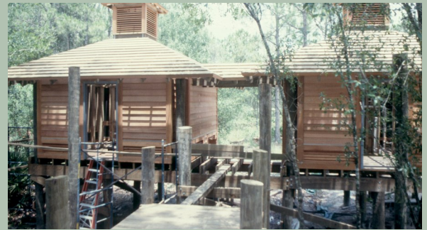
Outdoor Facilities under construction
