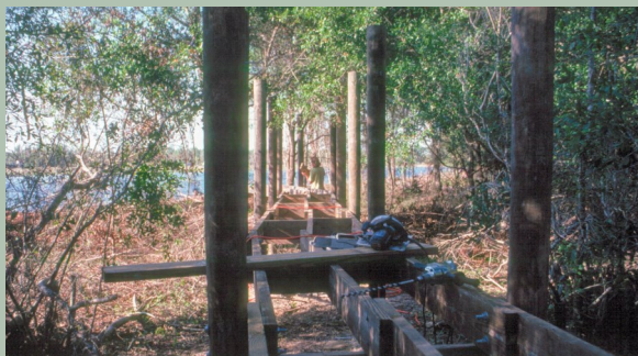
Building the "dock" along Gator Lake
