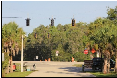
The traffic signal installation at the Slough entrance at Penzance Blvd.
